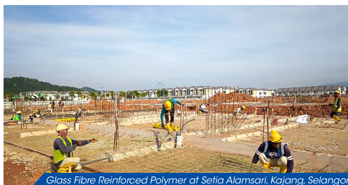
Glass Fibre Reinforced Polymer at Setia Alamsari, Kajang, Selangor
