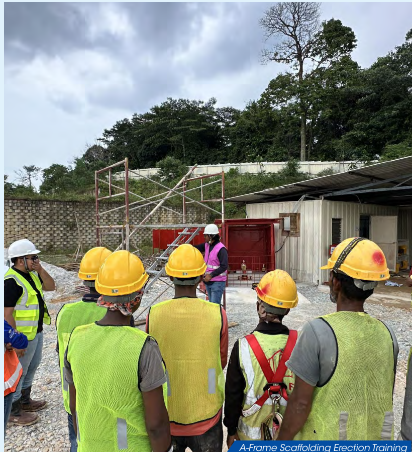
A-Frame Scaffolding Erection Training
