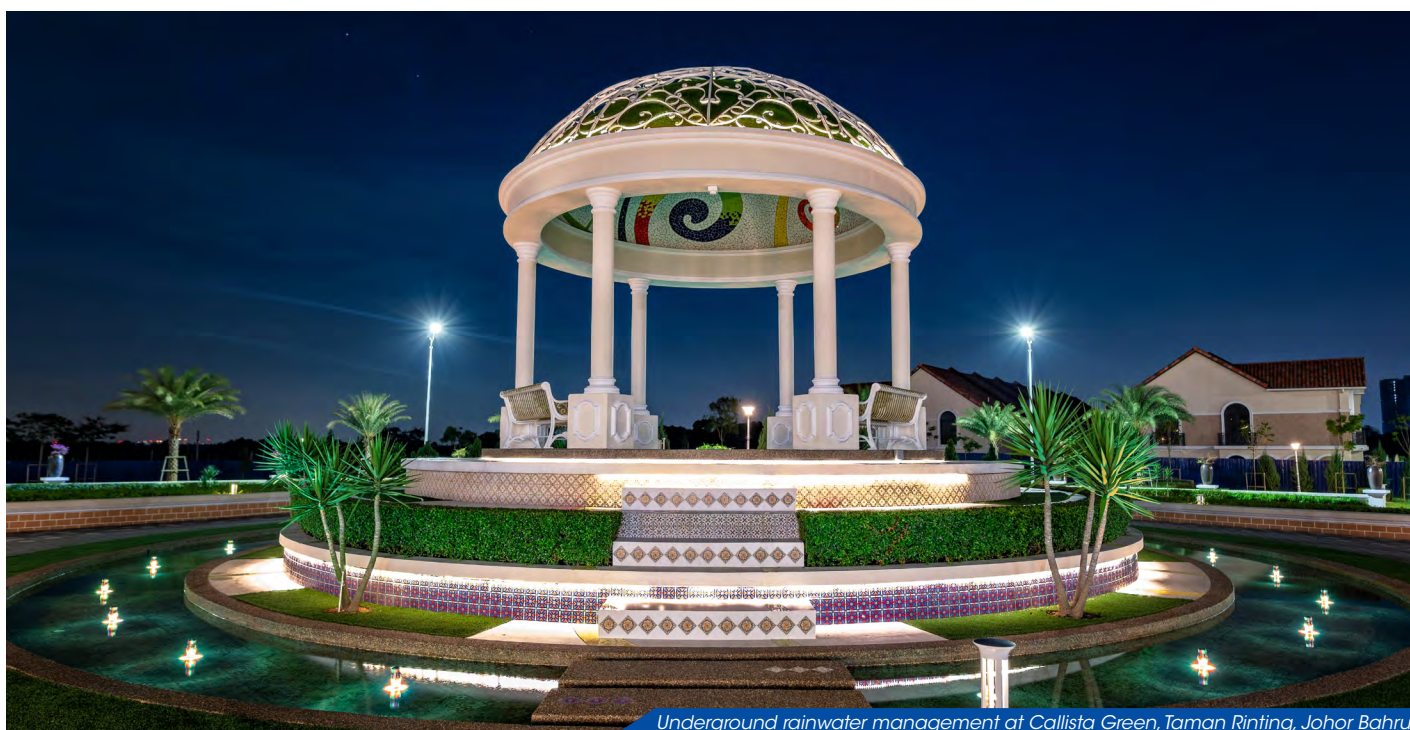
Underground rainwater management at Callista Green, Taman Rinting, Johor Bahru
