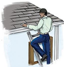
3. Make sure the gutter outlet / dome is clear from any debris that may clog the dome.
